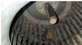
Dirty Fan Blades cause vibration and reduce the fan bearing lifetime.
