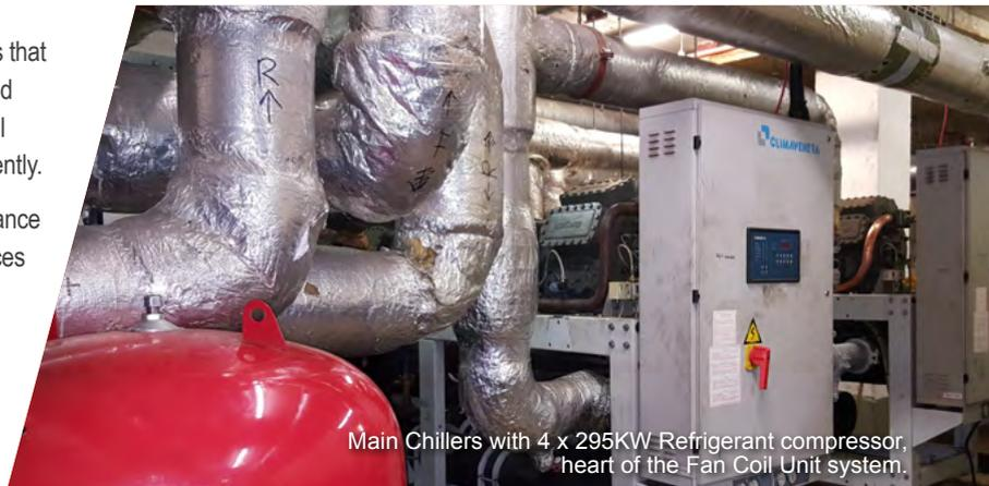
Main Chillers with 4 x 295KW Refrigerant compressor, heart of the Fan Coil Unit system.
