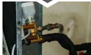
Upgraded/replaced valves and pipe insulation reduce risk of breakdown and condensation damage.
